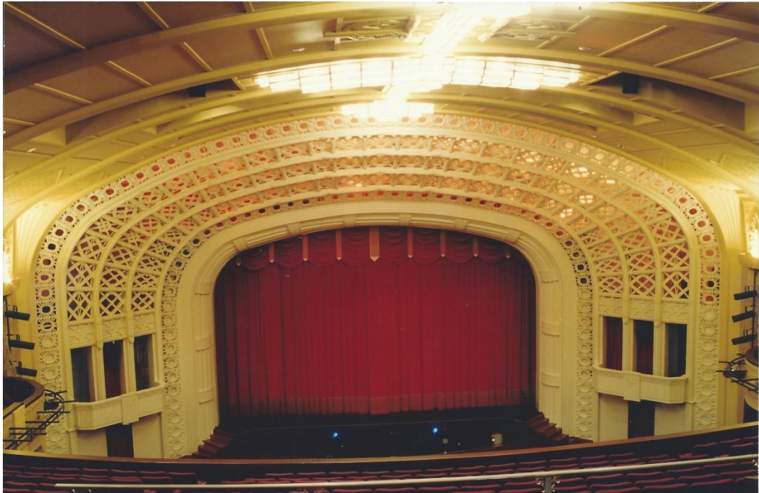
Toowoomba Empire Theatre fully restored after 20 years as a carpentry workshop for the local TAFE and now owned by Toowoomba City Council.
