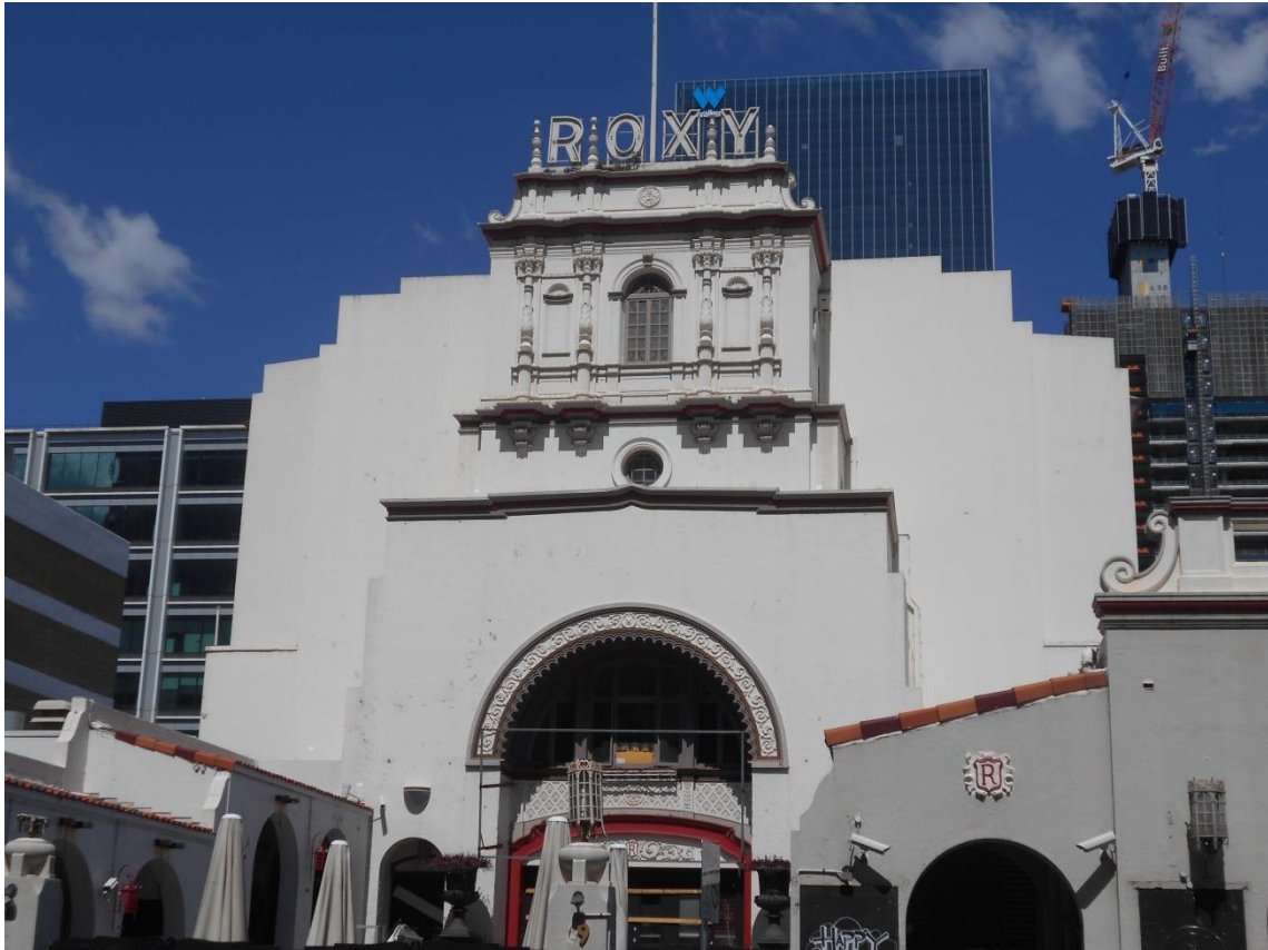
Even in its present state, the Roxy is still an awesome building. Photo: Les Tod
